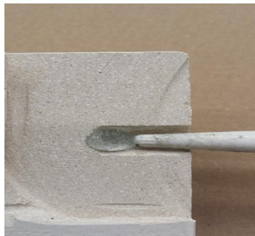
When adhesive is loaded in the two holes the tile is ready for installing, install the tile as shown on the photo to the right.
